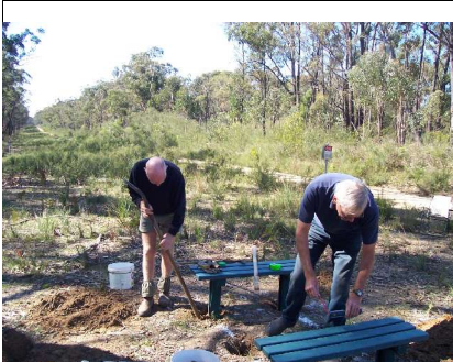
John and Michael measure things ready for installation.
