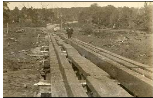
1914-15. Timbers have been laid across the piers but are not yet fastened in place.
